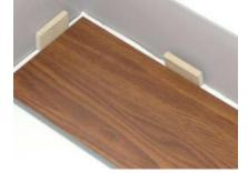
3. The end joints of the planks in the first row are assembled by inserting the tongue side into the groove side of the previous plank at a **natural angle**. Gradually lower the plank down flat until the end joint closes, ensuring that the planks are perfectly aligned. Install remaining full planks in the first row.
