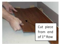
6. Install the long side of the first plank of the second row. Remember to place a 1/4" (6.3 mm) or 1/2" (12.7 mm) spacer between the wall and the short side of the plank. Insert the tongue side into the groove side of the previous row at a natural angle and rotate downward until plank is flat with the substrate. You should only have to lift the plank high enough to get your fingers underneath to achieve this natural angle
