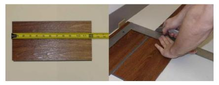
5. The remaining piece cut from the last plank in the first row may serve as the first plank in the second row provided it is at least 8" (20.3 cm) long. Always stagger end joints from row to row a minimum of 8" (20.3 cm).
