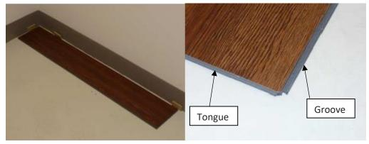
2. Place 1/4" (6.3 mm) spacers between the short and long side of the planks and the wall.
