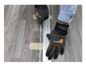
Place pieces of masking tape over seam edge to prevent movement. Using a sharp utility knife, doublecut through both pieces of flooring.
