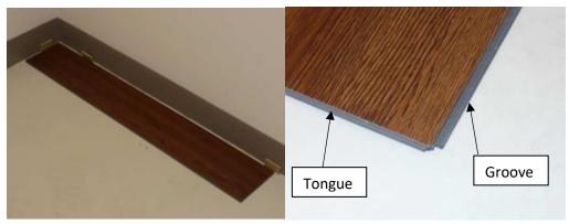
2. Place 1/4" (6.3 mm) spacers between the short and long side of the planks and the wall. Use 1/2" (12.7 mm) spacers for installations over both single wood construction subfloors and wood substrates that may be effected by moisture or external temperature and humidity fluctuations (i.e. crawlspaces, mobile homes).
