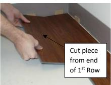
6. Install the long side of the first plank of the second row. Remember to place a 1/4" (6.3 mm) or 1/2" (12.7 mm) spacer between the wall and the short side of the plank. Insert the tongue side into the groove side of the previous row at a natural angle and rotate downward until plank is flat with the substrate. You should only have to lift the plank high enough to get your fingers underneath to achieve this natural angle
