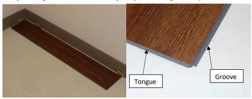
2. Place 1/4" (6.3 mm) spacers between the short and long side of the planks and the wall, use 1/2" (12.7 mm) spacers for installations over wood substrates that may be effected by moisture or external temperature and humidity fluctuations (i.e. crawlspaces, mobile homes)
