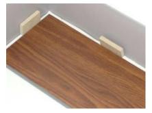
3. The end joints of the planks in the first row are assembled by inserting the tongue side into the groove side of the previous plank at a **natural angle**. Gradually lower the plank down flat until the end joint closes, insuring that the planks are perfectly aligned. Install remaining full planks in the first row.
