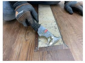
8. Prepare the replacement plank by removing the tongue and groove on each short side and by removing the groove on the long side.
