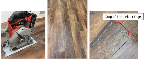
4. Carefully remove the center of the damaged plank.
