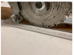
3. Carefully, cut the plank along the mark. Take care not to damage the adjacent plank. <u>CAUTION: wear the appropriate eye protection</u>, respiratory equipment and be certain that the safety guards are in place and operational
