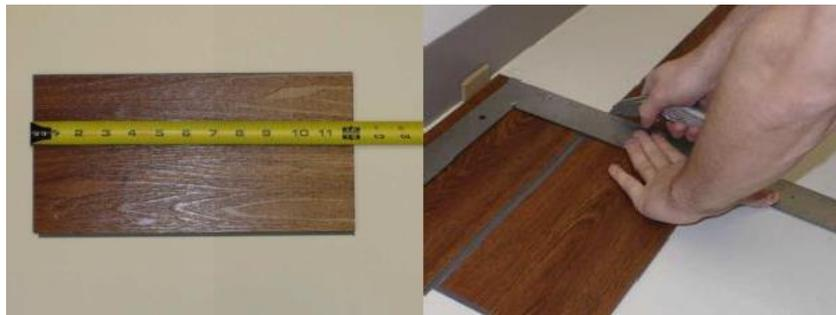
5. The remaining piece cut from the last plank in the first row may serve as the first plank in the second row provided it is at least 12" (30.4 cm) long. Always stagger end joints from row to row a minimum of 12" (30.4 cm).
