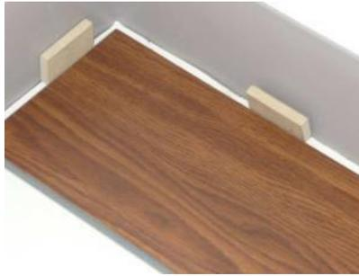
3. The end joints of the planks in the first row are assembled by inserting the tongue side into the groove side of the previous plank at a **natural angle**. Gradually lower the plank down flat until the end joint closes, insuring that the planks are perfectly aligned. Install remaining full planks in the first row.
